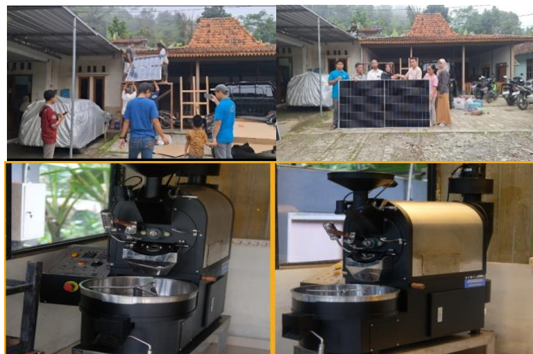
Figure 4. Installation of solar panels and coffee roasting equipment
