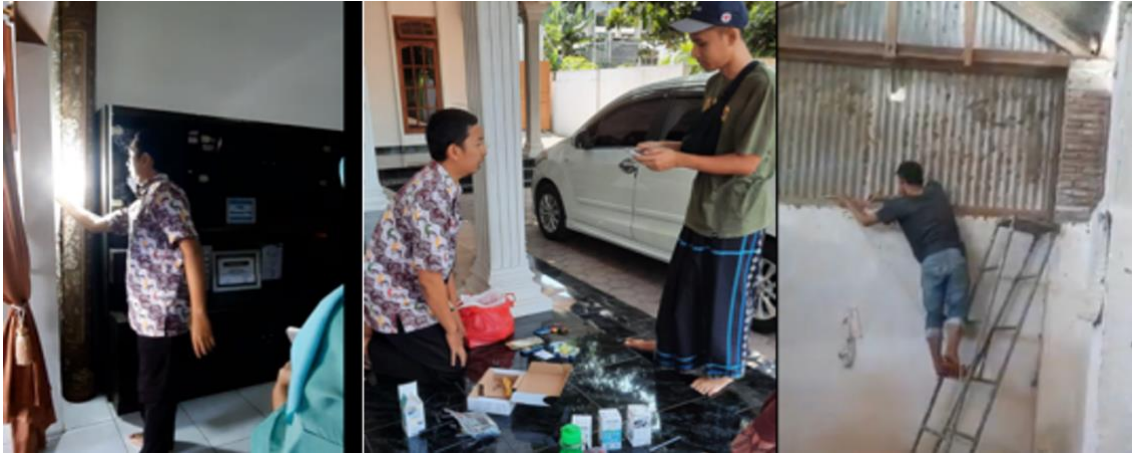
Gambar 4. Proses instalasi hardware dan software kontrol lampu
