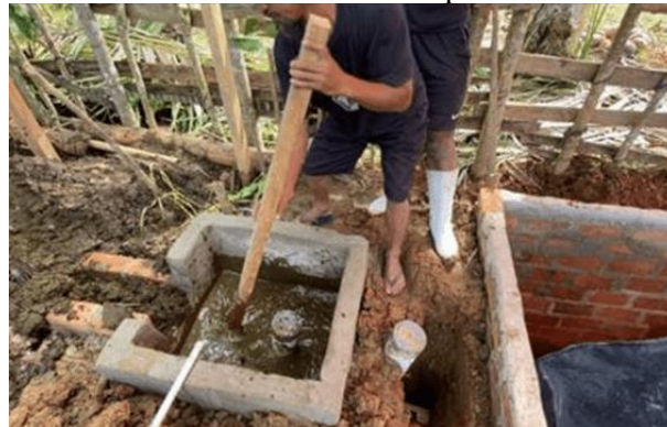
Gambar 8. Proses pengisian digester
